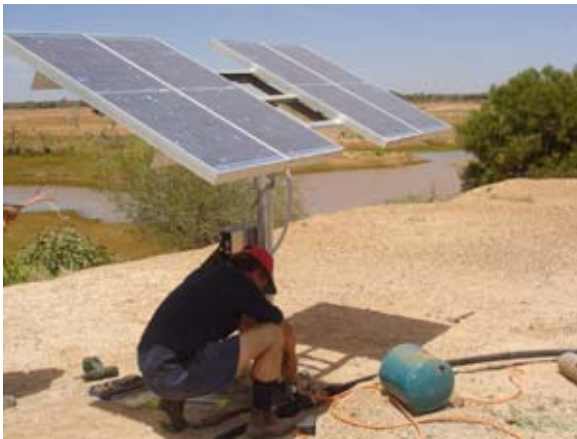
Chris Blackmore installing solar panels at Gypsum Dam
